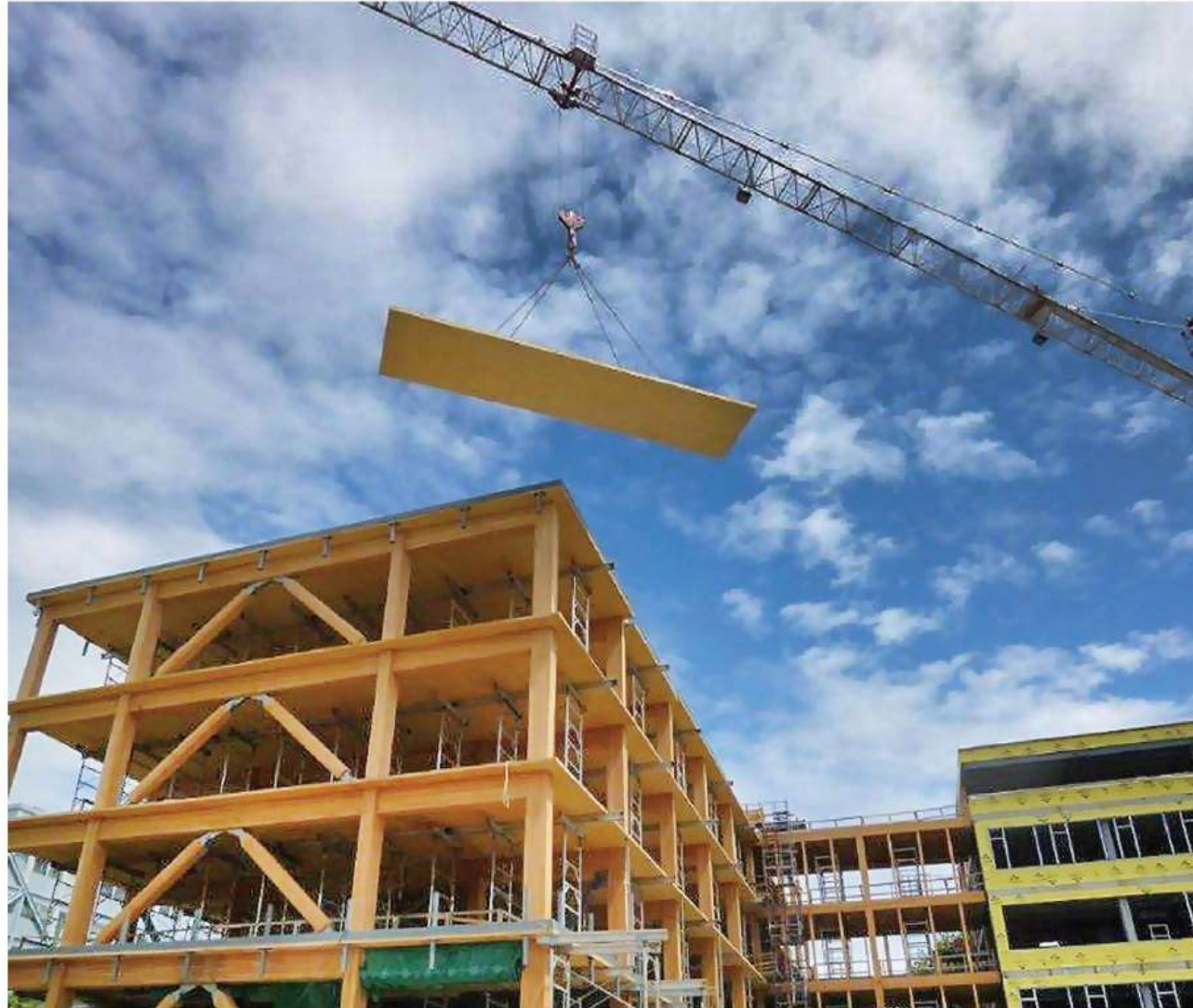
A COMPOSITE LAMINATED TIMBER PANEL BEING CRANED INTO PLACE.
