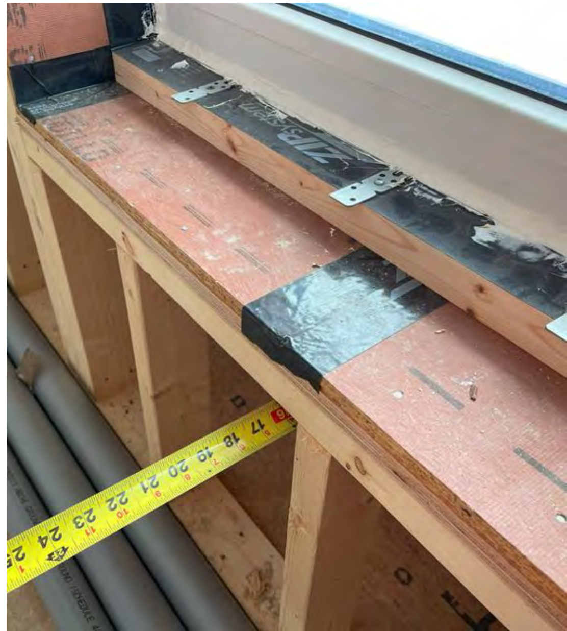
Image: Airtight Engineering
