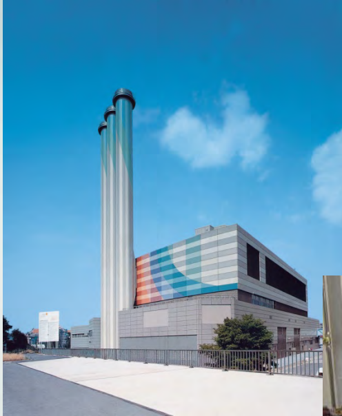
District Heating 260MW e
